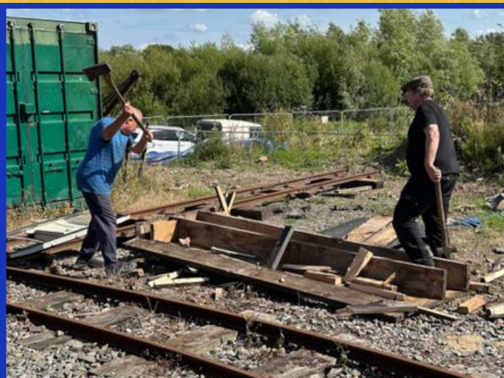
Gordon and Dave demonstrate their specialist skill - demolishing things.
