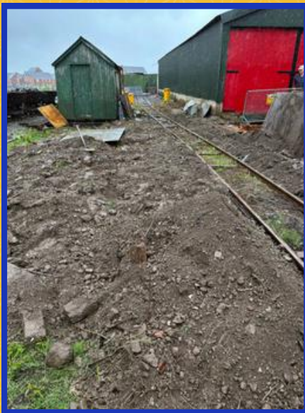
The end result - a well-supported section of track. Still raining.
