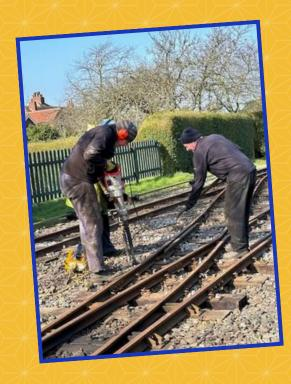
The track near the station also gets some attention, packing ballast under a replacement sleeper.
