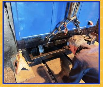
Mike slides the new bogie into place, with help from Alan on the hoist controls.
